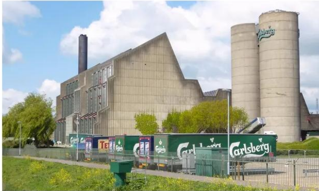
📍 The Carlsberg brewery in Northampton where an industrial accident caused an ammonia leak. Photograph: Google Maps
